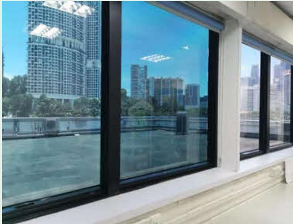
Climate change has resulted in rising temperatures during the day. Lowering temperature setpoints are required to maintain the ambient temperature in the laboratory for keeping laboratory equipment at optimum performance. **Pharmaceutical Laboratory** has implemented temperature mitigation measures through the installation of solar films on windows, improving the temperature setpoint by 2°C.
